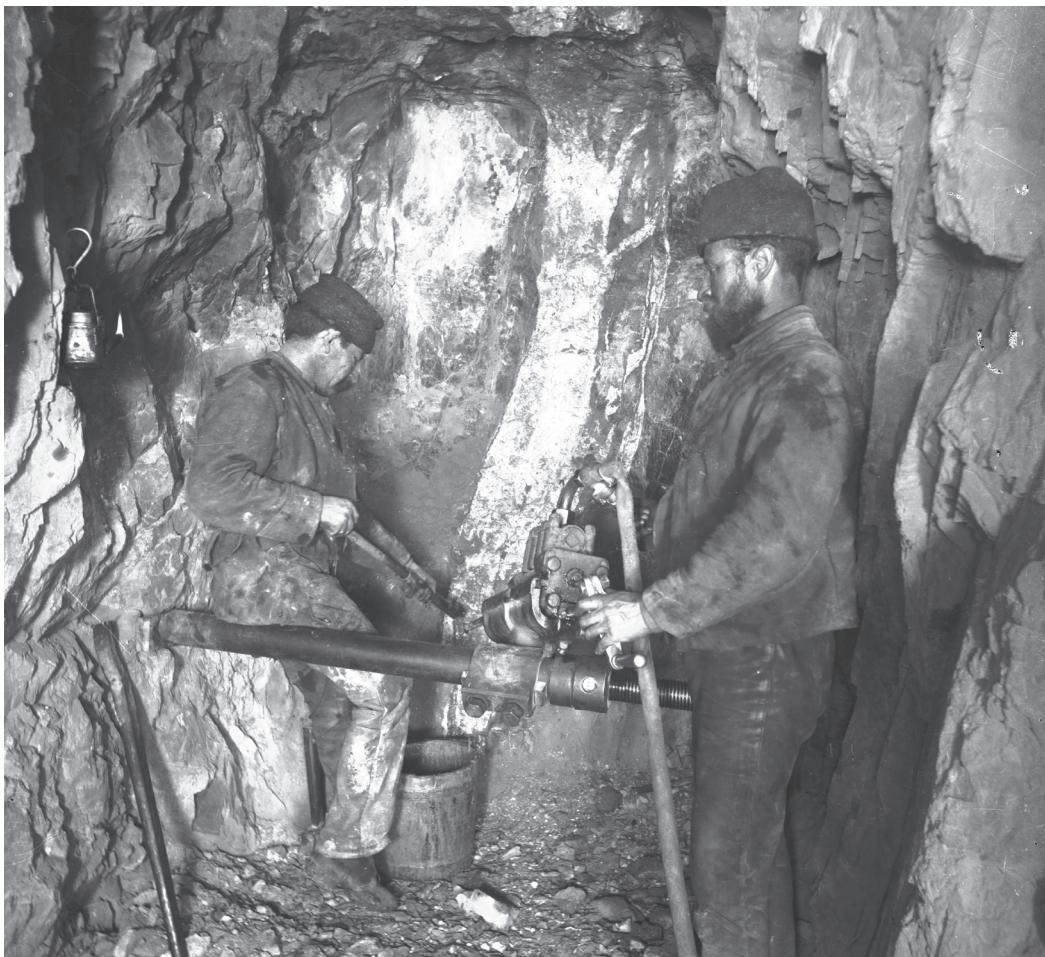
Figure 9: On location The narrow ore vein is worked with a pneumatic jackhammer.
